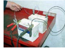
Connecting batteries in parallel (12 V)
