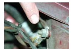
Earth or ground cable
