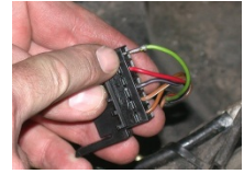
Damaged wiper motor connections
