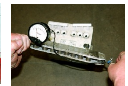
Battery heavy duty discharge test
